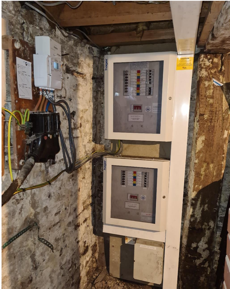
Figure 5 - Distribution Boards
