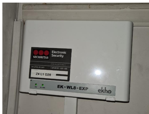
Figure 16 - Wireless Expander Module
