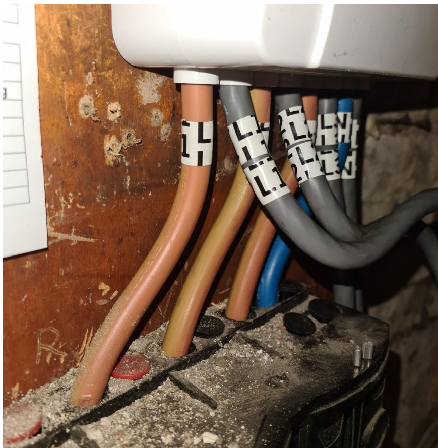
Figure 4 - Degradation of cable insulation below meter
