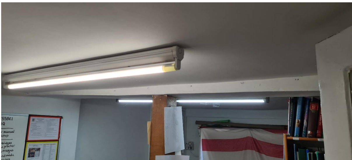
Figure 9 - Example of surface mounted batten fitting
