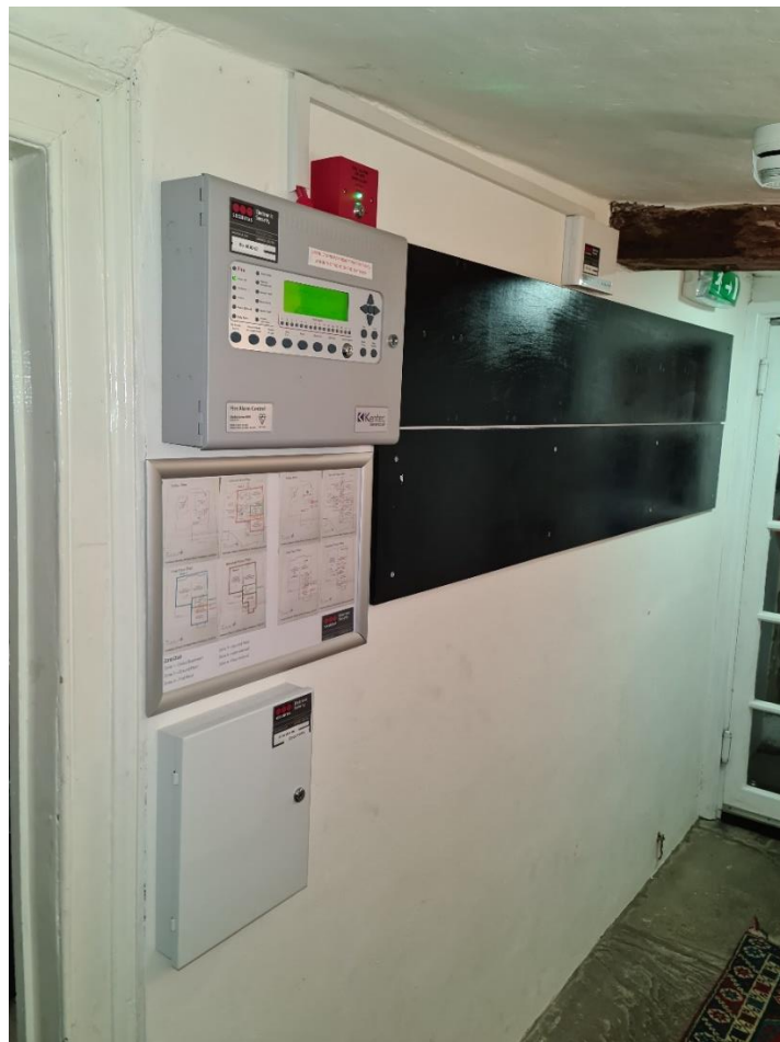
Figure 13 - Fire Alarm Control Panel, Zone Plan & Logbook
