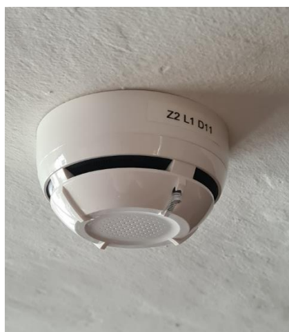
Figure 15 - 3-in-1 Optical Smoke Detection
