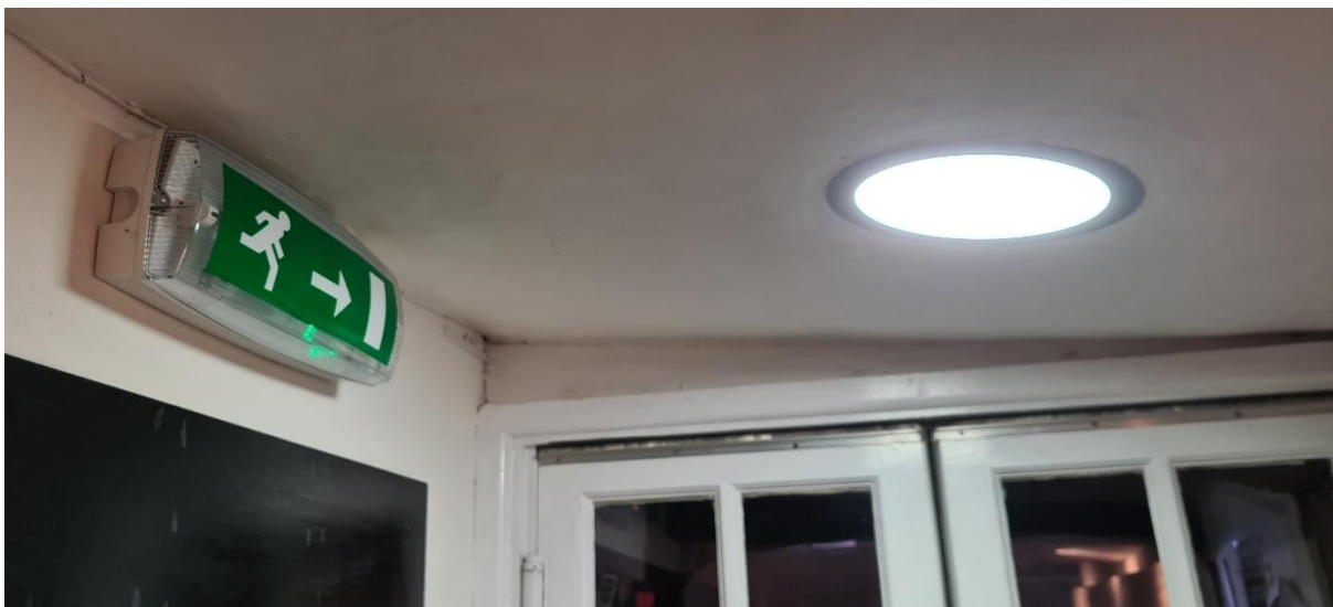
Figure 8 - Example of emergency bulkhead and recessed LED fitting
