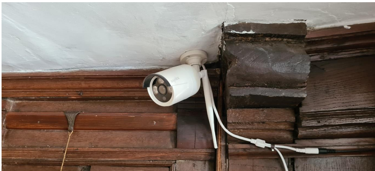
Figure 18 - Wireless CCTV Camera
