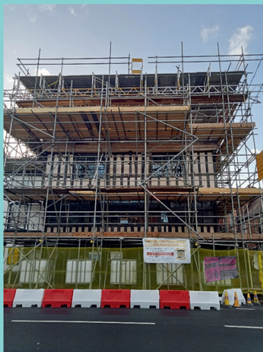
The scaffolding completely surrounds the building.
