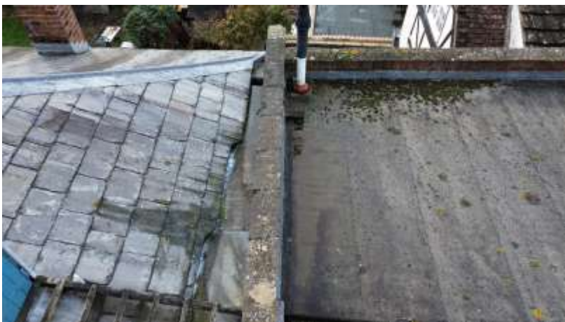
North parapet main hall
