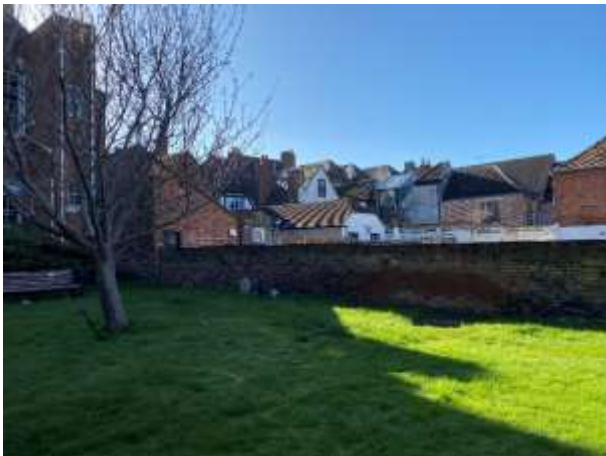
Gardens south boundary wall.
