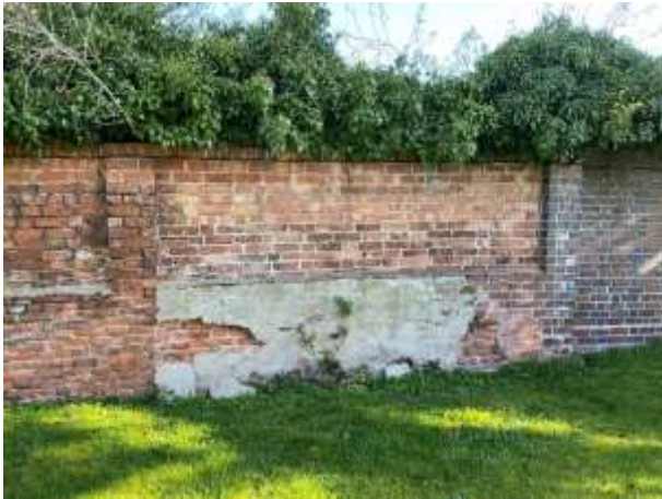
Gardens north boundary wall.
