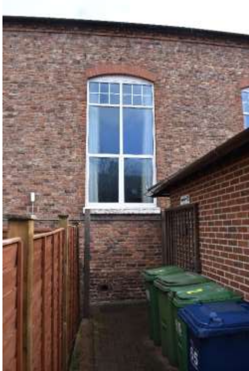
West Wall of Main Hall
