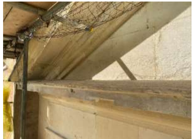
Corn exchange east wall stone repair in progress.
