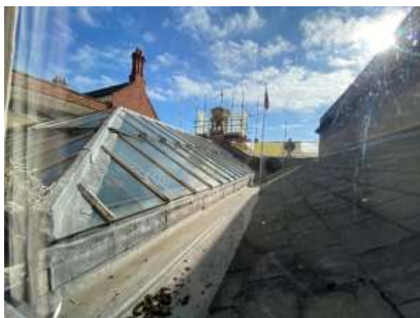
Corn Exchange south aisle roof.
