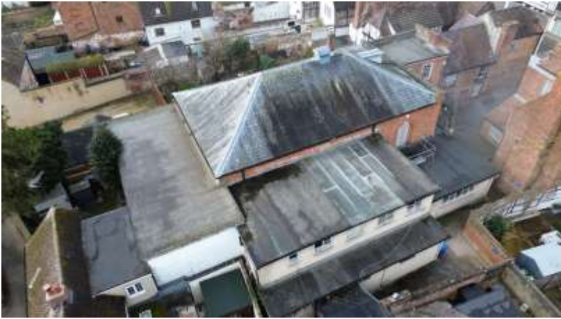
Roofs from east
