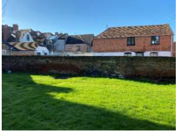
Gardens south boundary wall.
