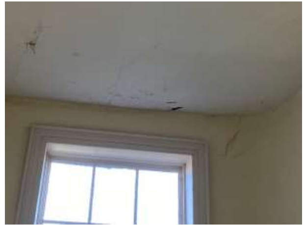
Town Hall stairwell ceiling.
