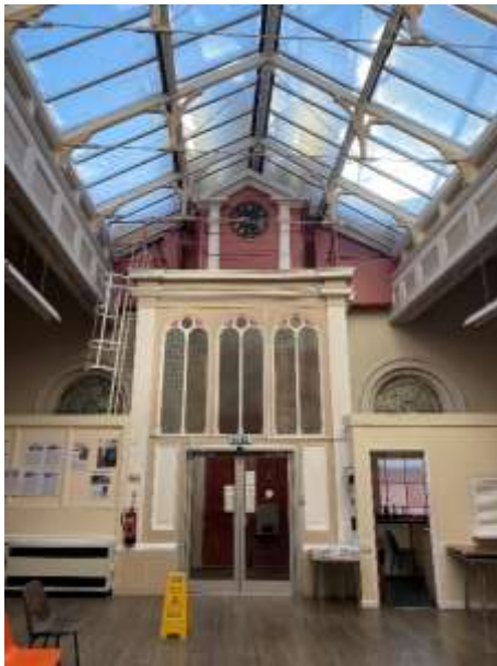
Corn Exchange east wall.
