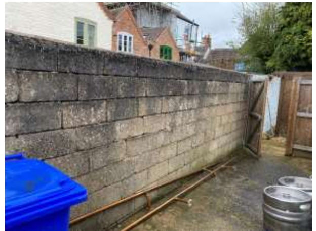
Boundary wall to north of cold-store
