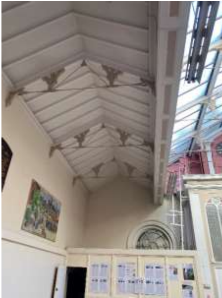
Corn Exchange north aisle roof.
