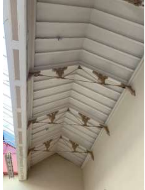
Corn Exchange south aisle roof.
