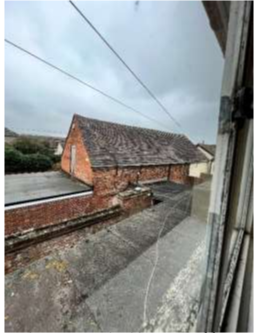
Tudor Room and cold-store roof from west
