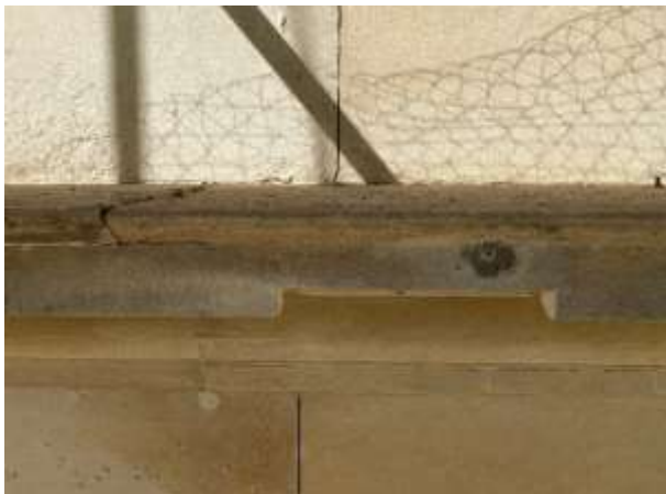
Corn exchange east wall stone repair 2 in progress.
