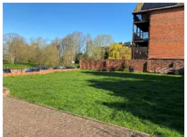
Gardens north boundary wall.
