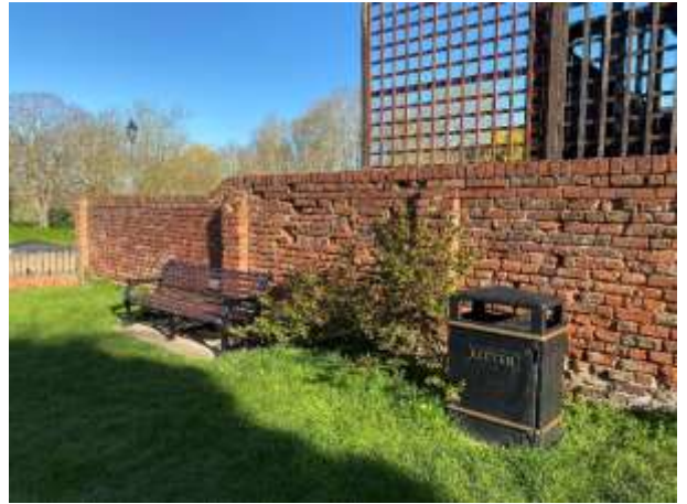
Gardens north boundary wall.
