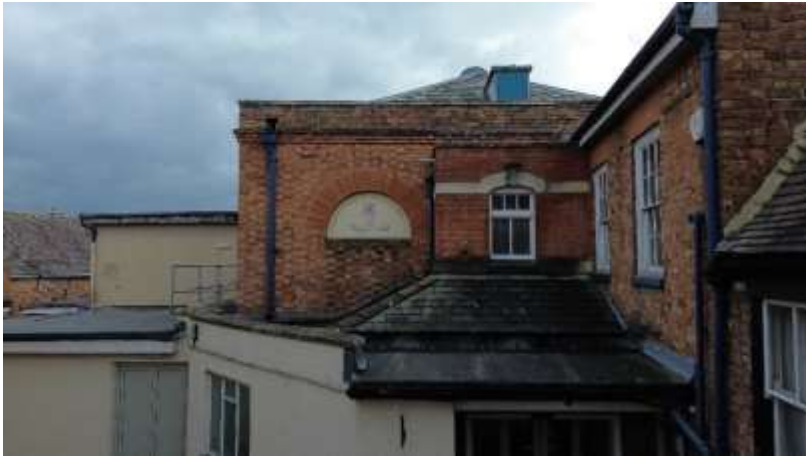
Roof from north
