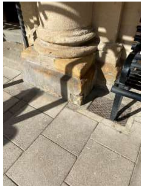
Column base right-hand side of entrance doors.
