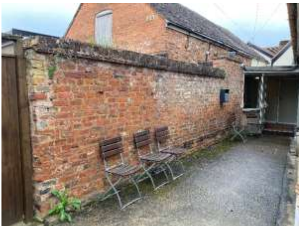
Brick wall between cold store and WCs
