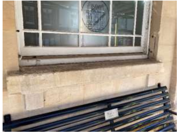
Corn Exchange east wall window cill.
