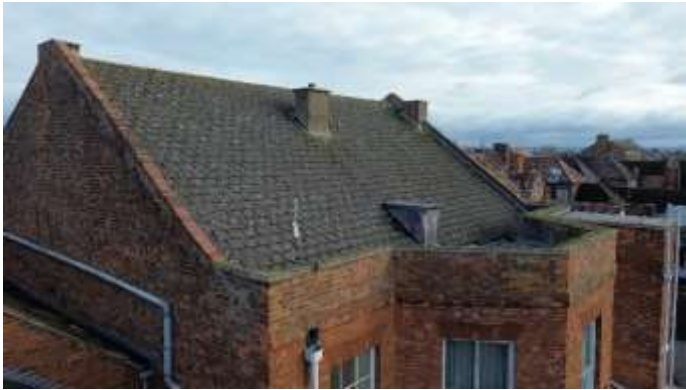
Town Hall roof west slope.
