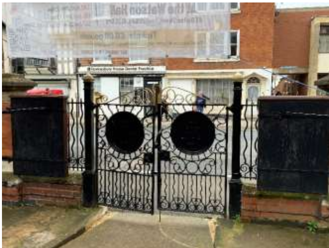
Entrance gates off High Street
