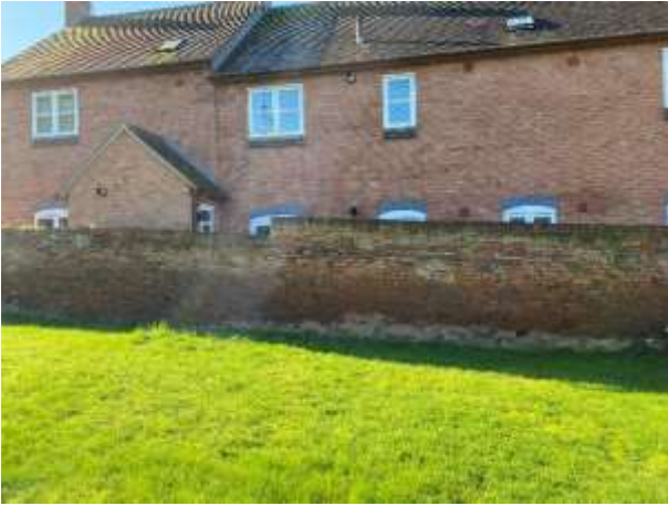
Gardens south boundary wall.
