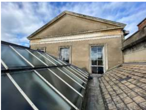
Town Hall east wall.
