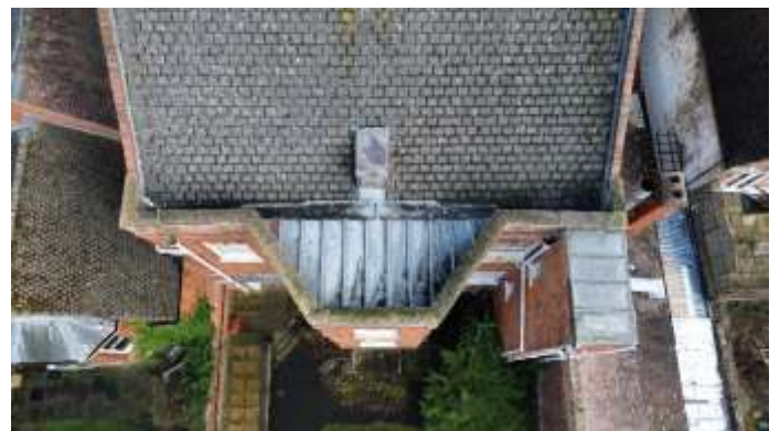
Town Hall roof west slope and bay.
