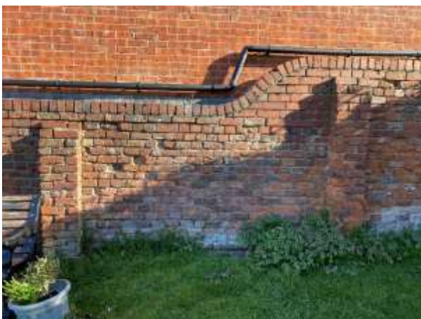
Gardens north boundary wall.
