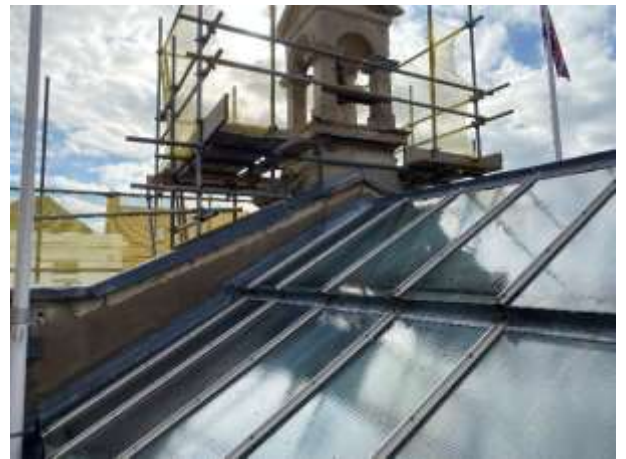
Corn Exchange roof east end and bellcote.
