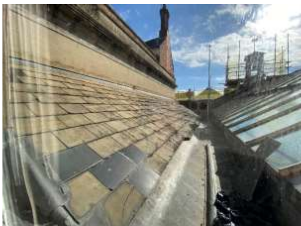
Corn Exchange north aisle roof.
