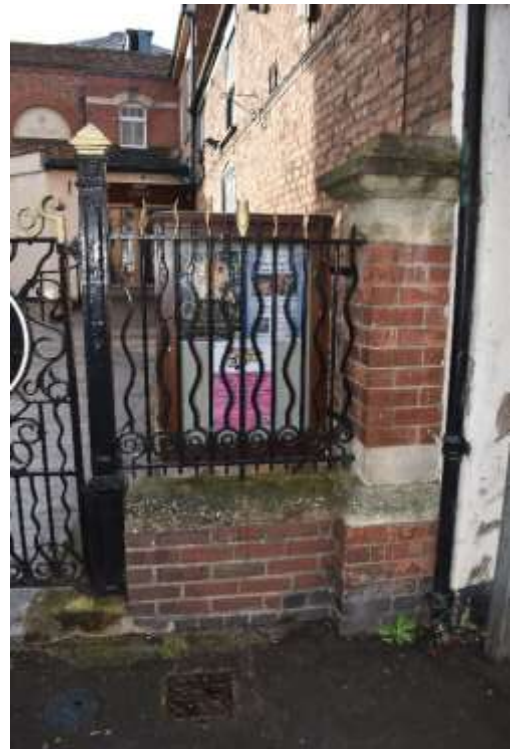
Entrance gates railing and brick pier
