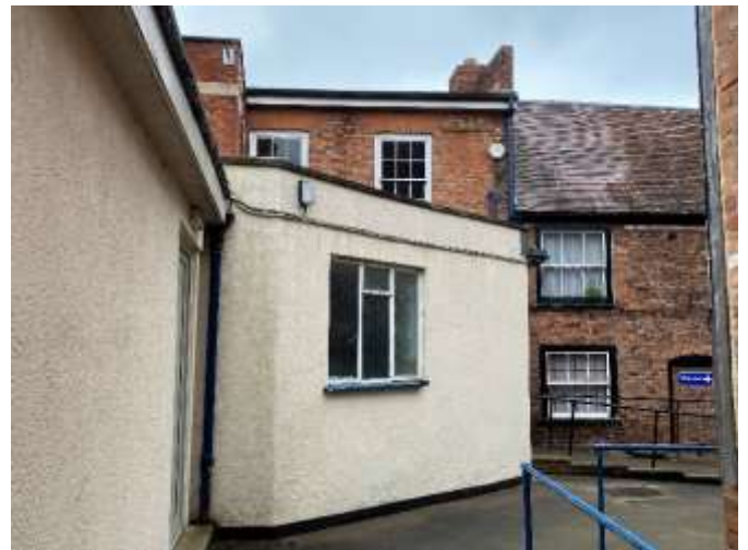
East wall of Foyer
