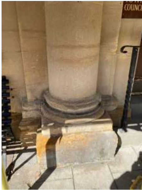
Column base left-hand side of entrance doors.
