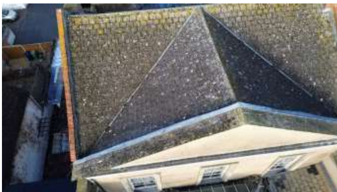
Town Hall roof east slope.
