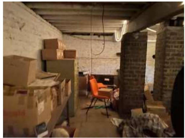
Basement under Corn Exchange.
