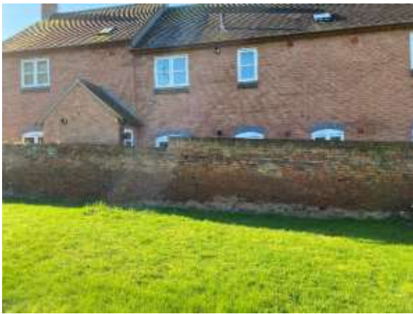
Gardens south boundary wall.
