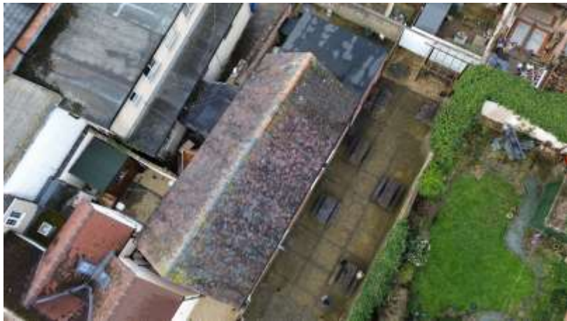
Tudor Room roof from south-east
