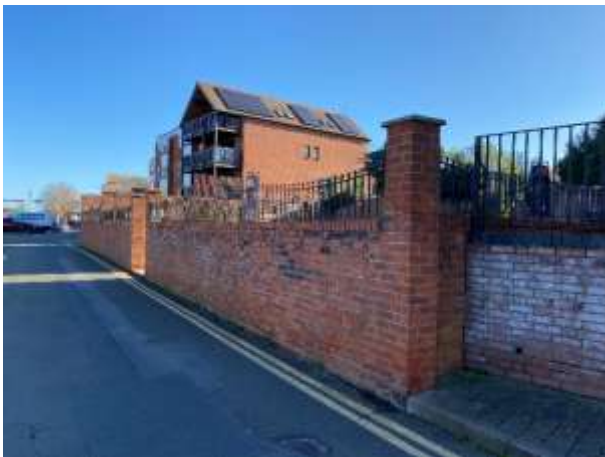
Gardens west wall.
