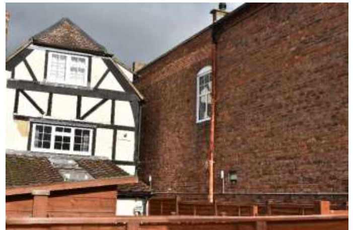
West wall of Main Hall
