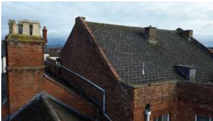
Town Hall north wall.
