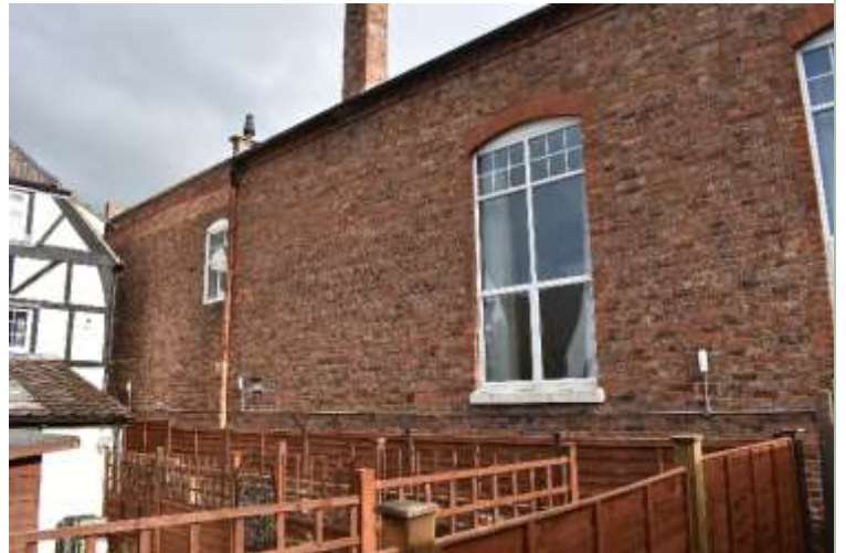
West Wall of Main Hall
