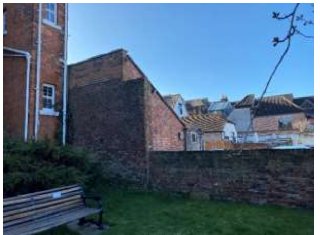
Gardens south boundary wall.
