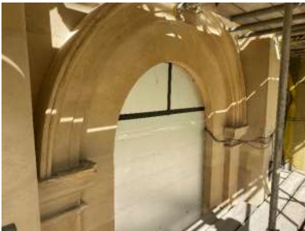
Corn Exchange east wall window head.
