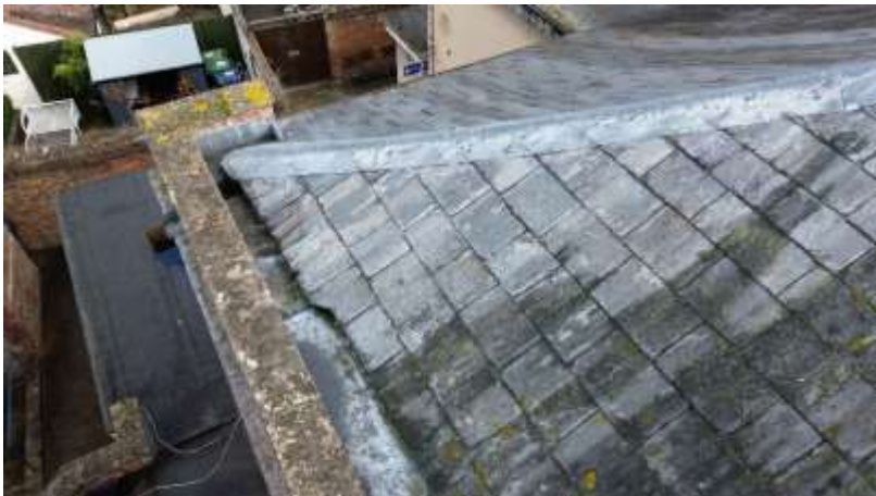
North parapet main hall
