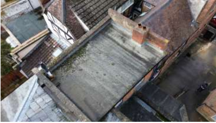
Stairwell roof from south
