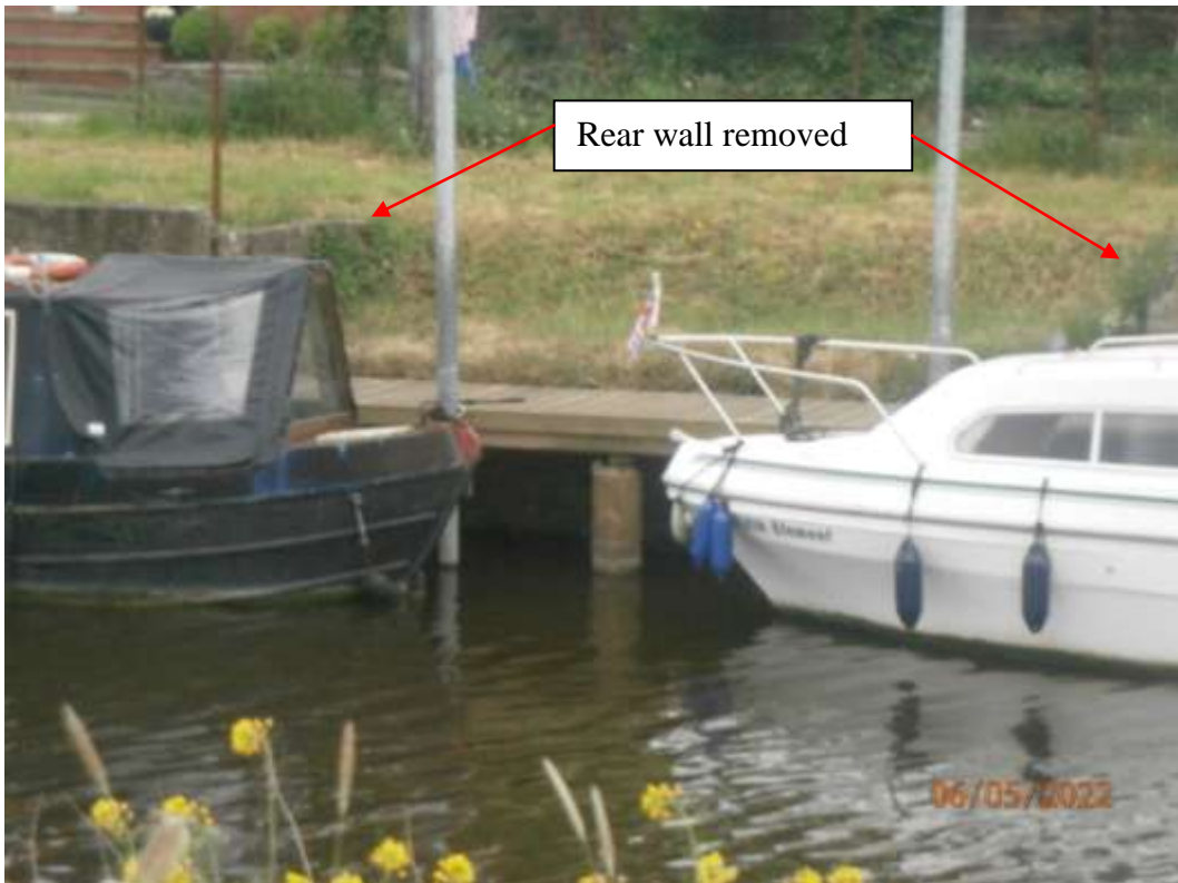
Original Landing – Rear wall removed & grassed to wall front edge
