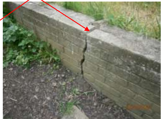
Vertical Crack
