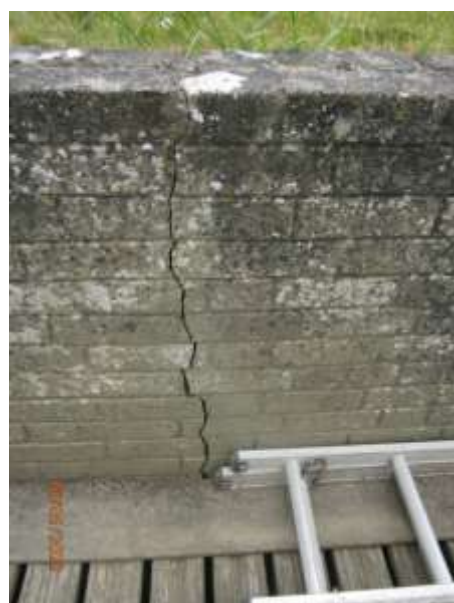
Crack mid-length
