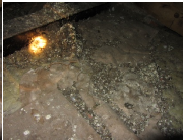
Internal guttering. Prone to blockage by guano from the many pigeons
