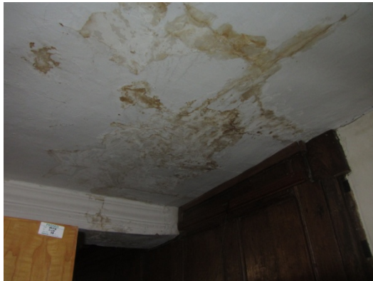
Ceiling 1 st Floor Water ingress above battlefield gallery (being refurbished for 550 th anniversary)
