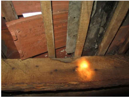
Roof. Various holes, slipped tiles, bowed beam indicating movement
