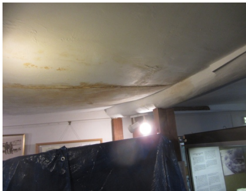
Ceiling 2 nd Floor Water damage above WW1 display
