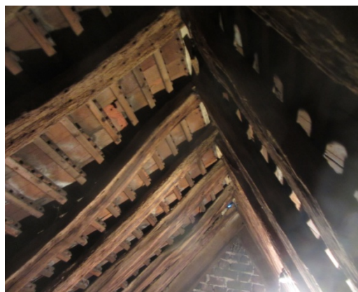
Ceiling 2 nd Floor above old fair display Roof. No lining
