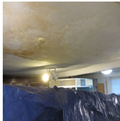
Ceiling 1 st Floor Water ingress above battlefield gallery (being refurbished for 550 th anniversary)
