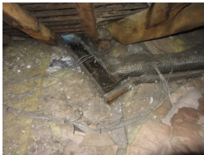
Internal guttering. Prone to blockage by guano from the many pigeons
